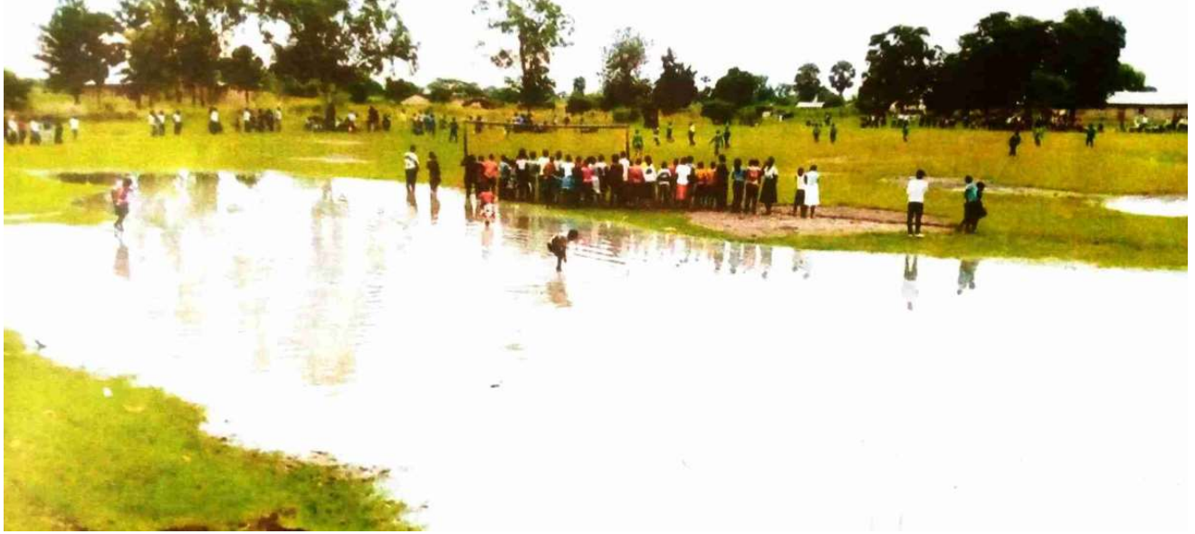
FLOODED SCHOOL DUE TO POOR DRAINAGE CONSTRUCTION OF THE ROAD –REQUESTED FOR ROAD REDESIGNING AND DRAINAGE SYSTEMS CHANGE TO AVERT THIS HAZARD.
